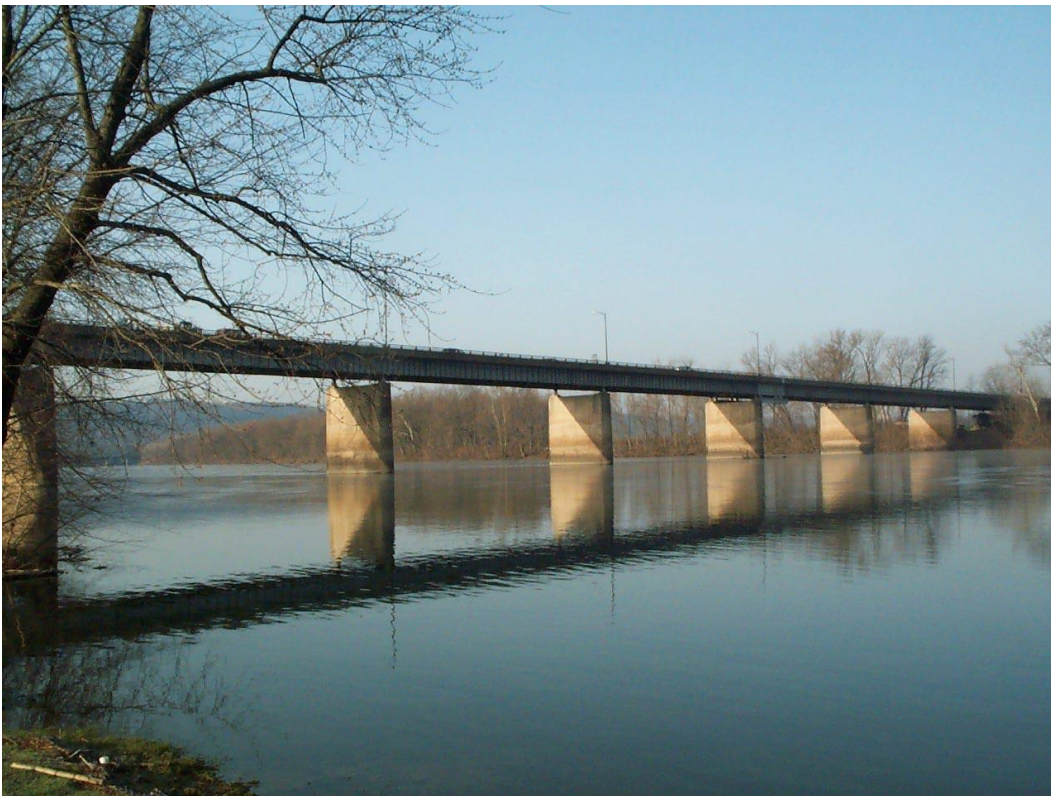
Figure 3 – Muncy/Montgomery River Bridge Over The Susquehanna River
